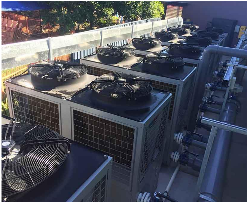
Figure 5 Multiple heat pump installations at Dreamworld Gold Coast Qld
