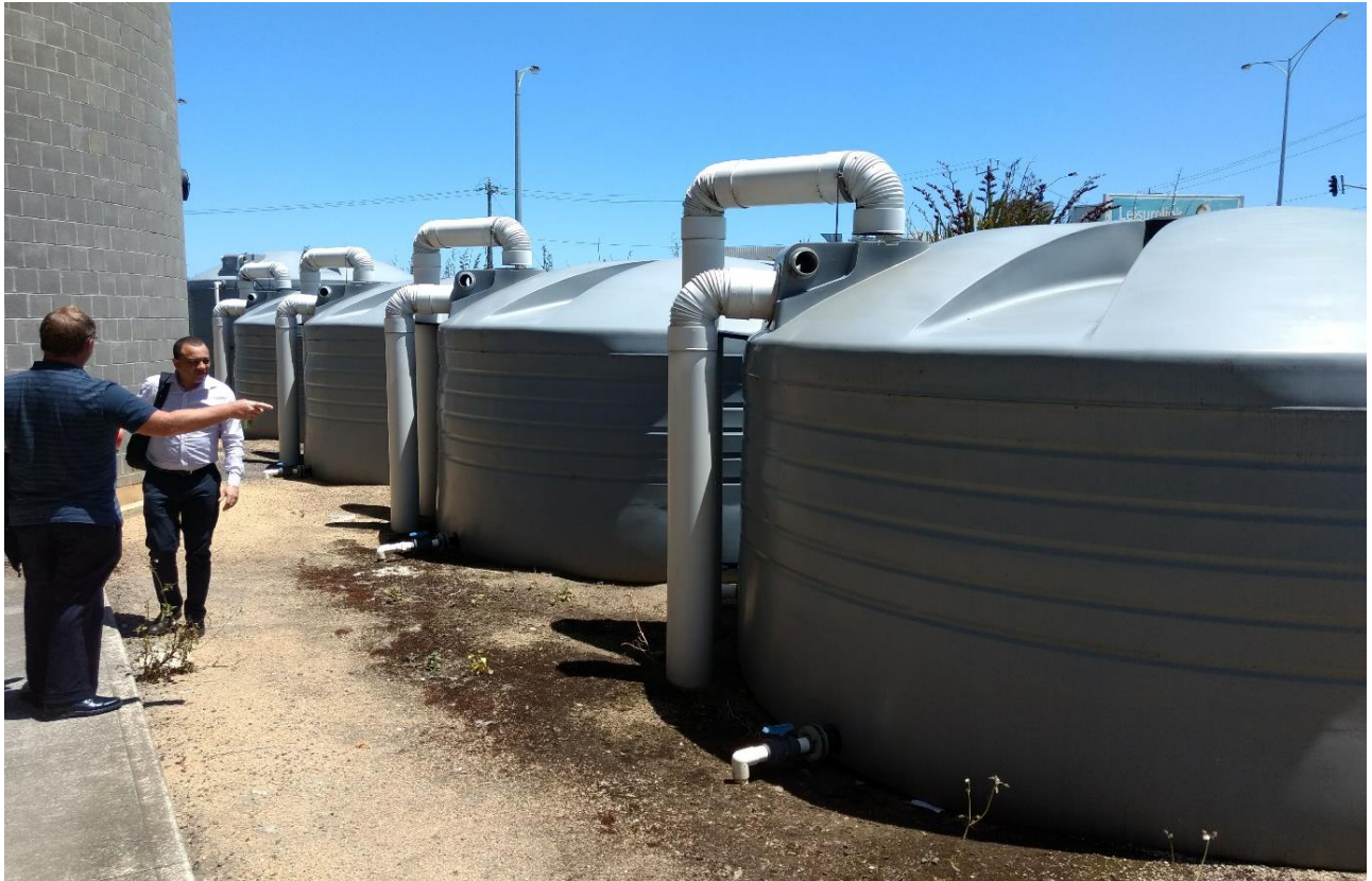
Figure 9: 30,000L water storage tanks at LeisureLink Geelong
