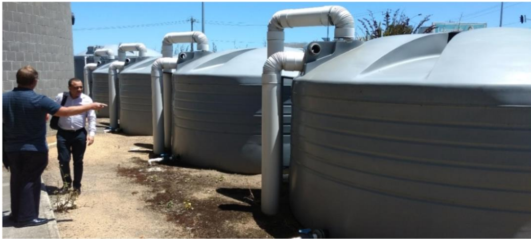
Figure 14: 30,000L water storage tanks at Leisure Link, Geelong
