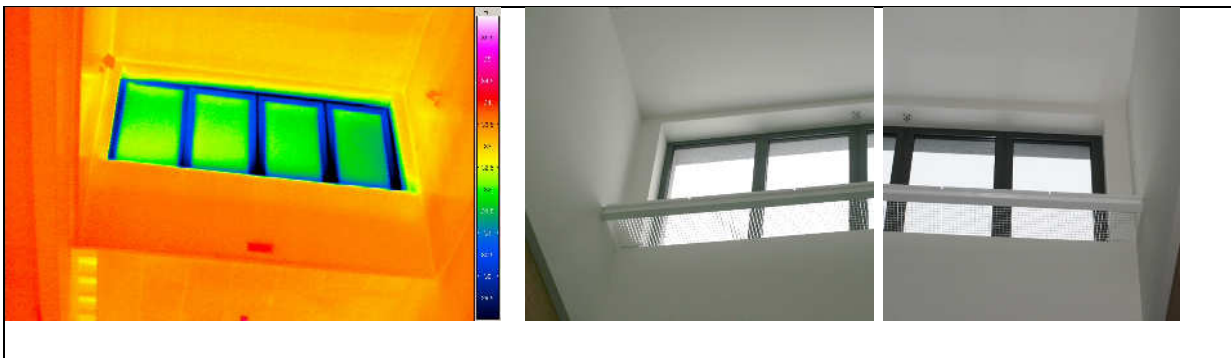
Figure 43: View of a roof shed with glazing (Shed) with a grate for maintenance;
