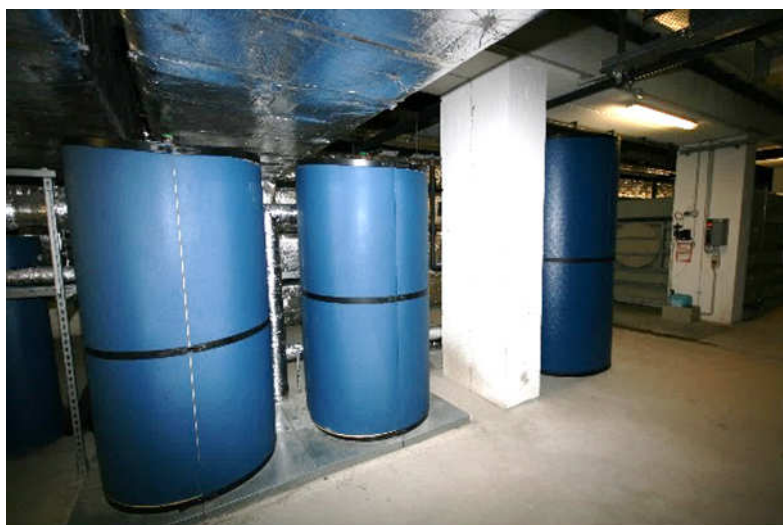
Figure 89: Three thermally insulated hot water tanks
